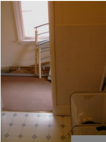
Wall Finish, Skirting, Light Switch
