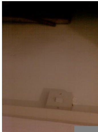
All Walls in Room
