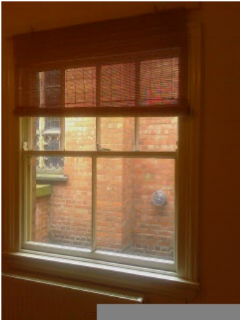
All Windows in Room, Blind (roller), Window glass
