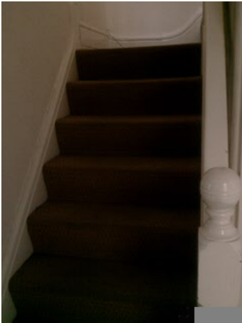
Stairs, Stairs Floor, Handrail, End Post, Stair Riser, Stair Tread
