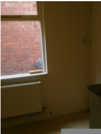
Painted plaster front wall, Wall Finish, Skirting, Light Switch (double)
