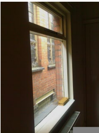
All Windows in Room, Window frame/sill, Window glass
