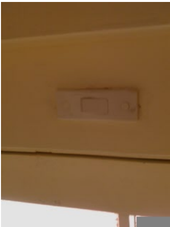
All Walls in Room, Wall Finish, Light Switch (single)
