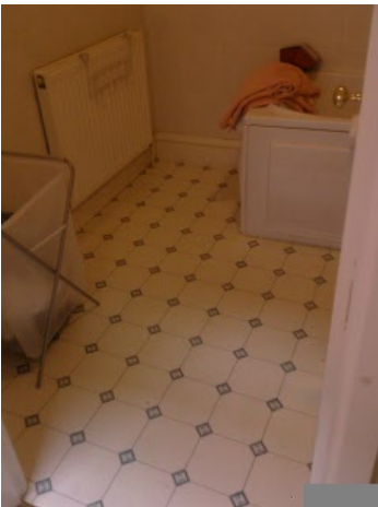
All Flooring in Room
