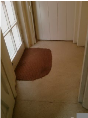
All Flooring in Room
