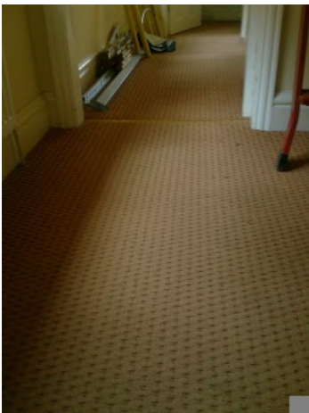
All Flooring in Room
